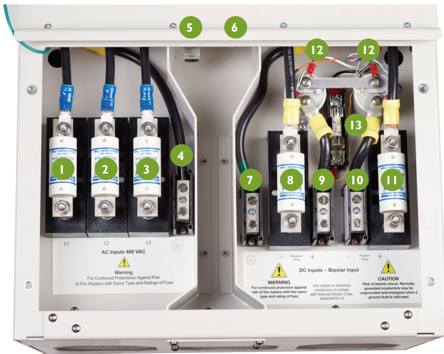
Figure 3. Inverter Wiring Compartment
